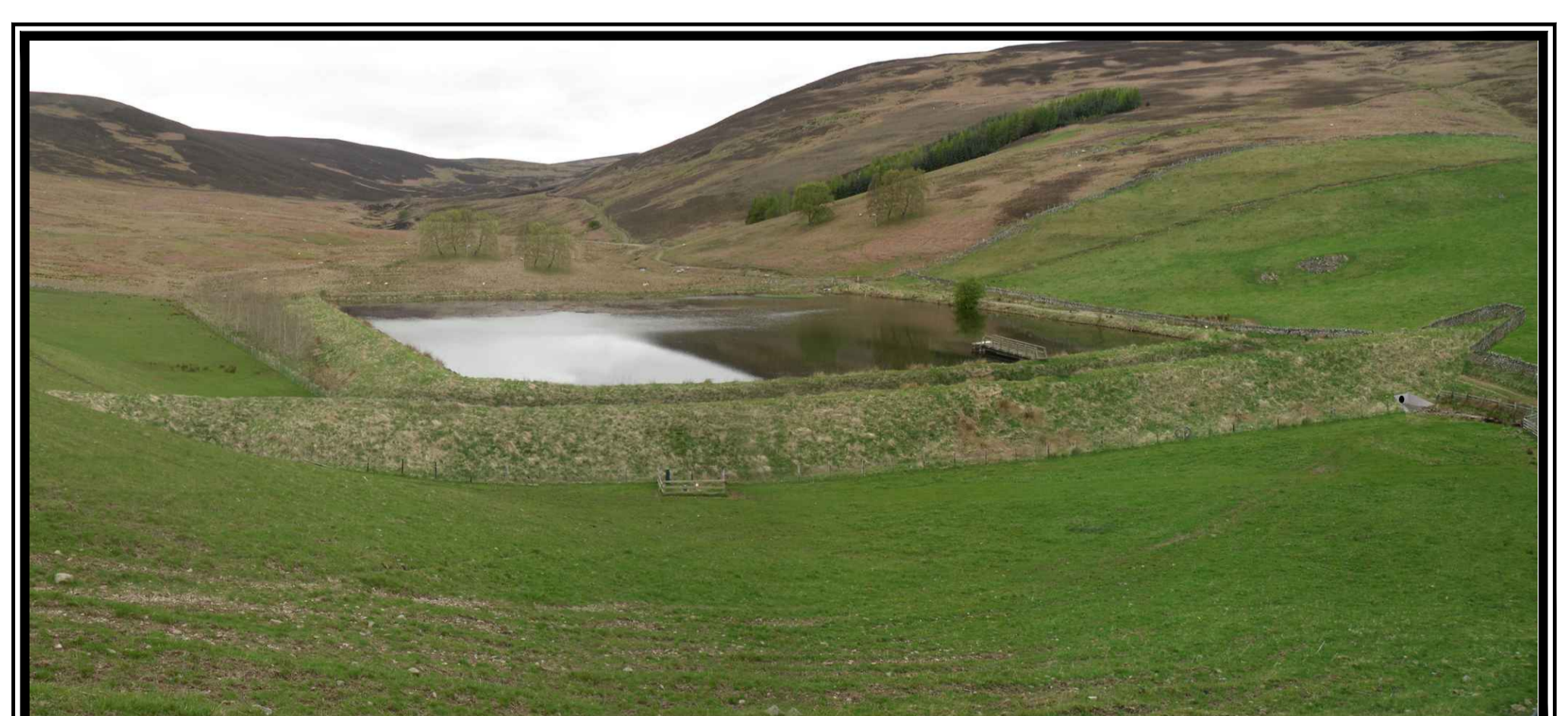
Utilisation of flood storage to reduce flood impact of Long Philip Burn
